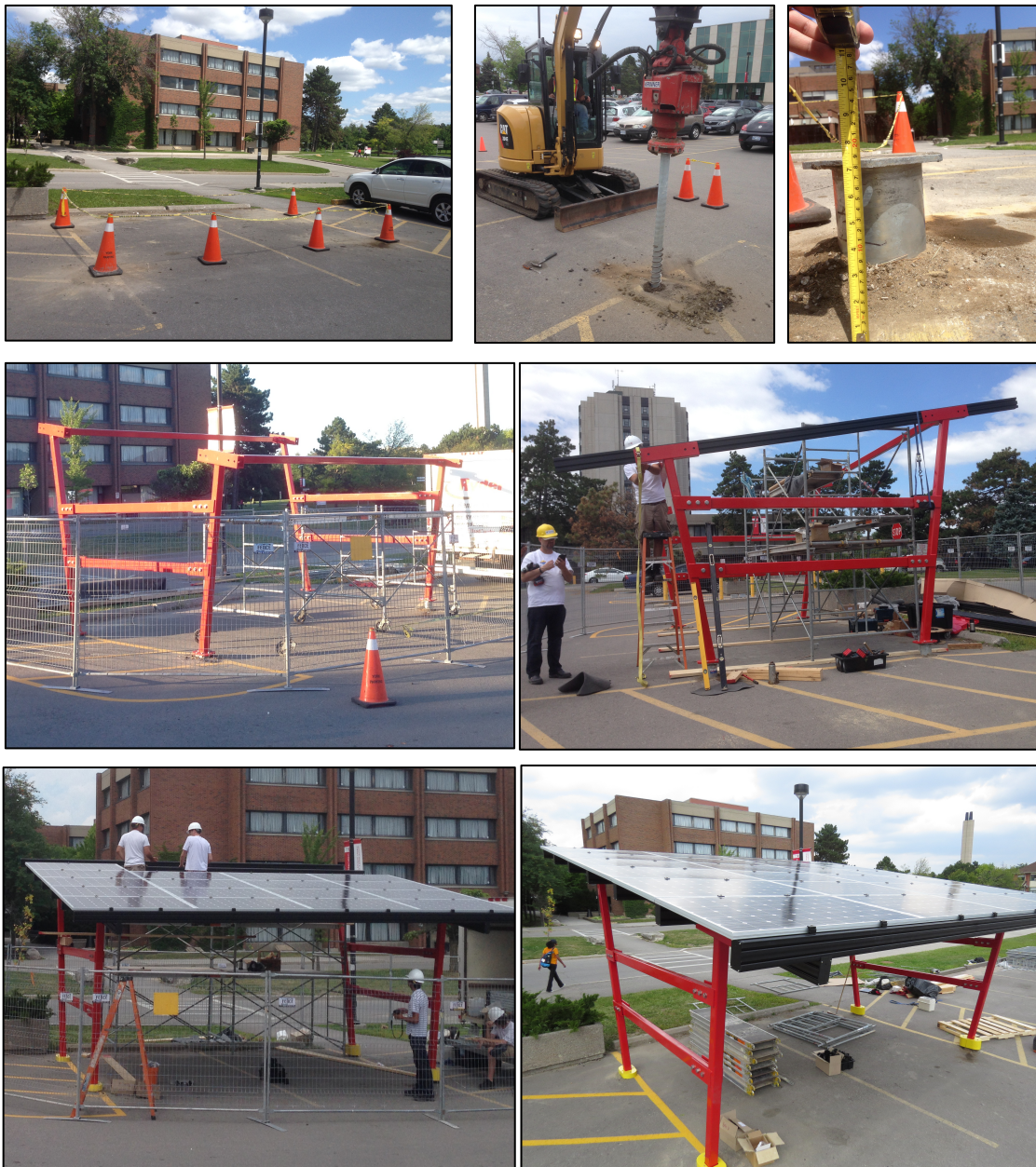
Figure 9: Photo sequence of REM structure installation. Photo Source: Mustafa Nazari
