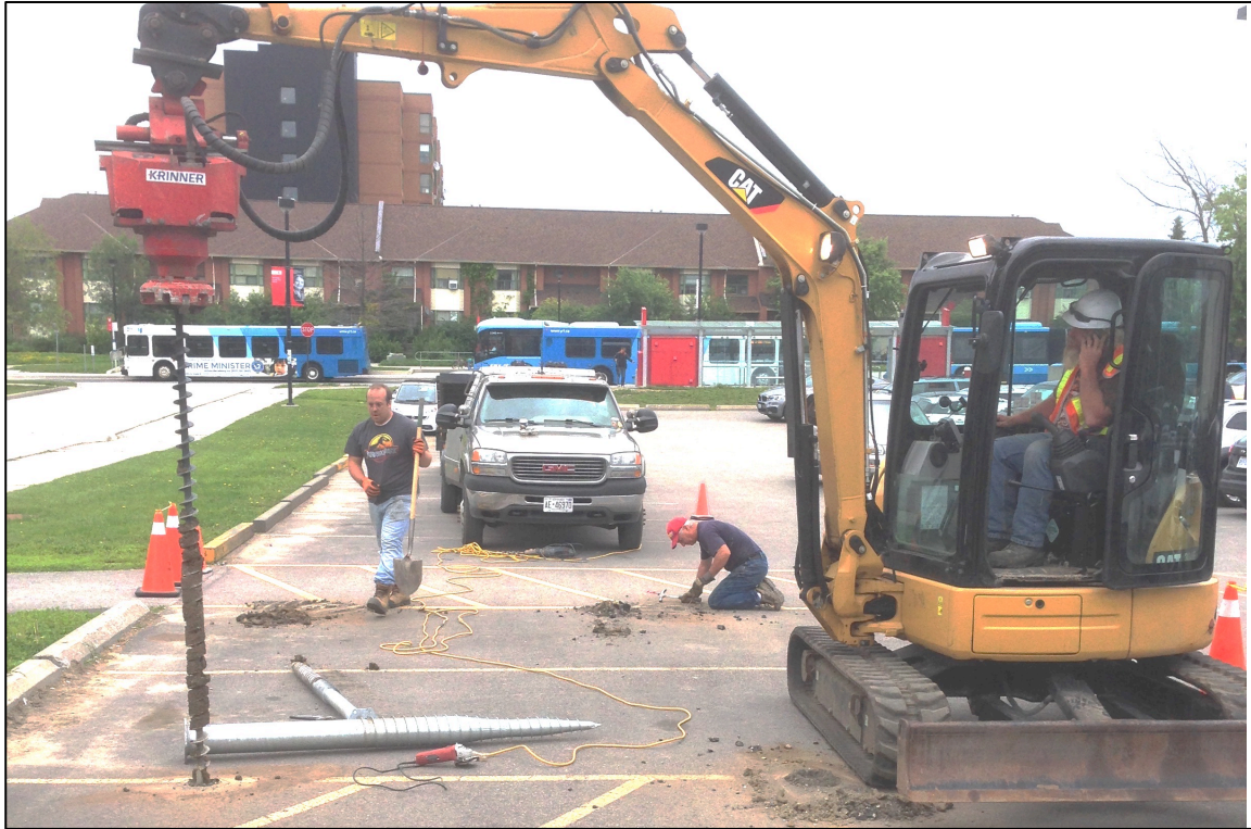
Figure 7: KR B 40 driver pre-drilling pilot hole. Photo Source: Mustafa Nazari
