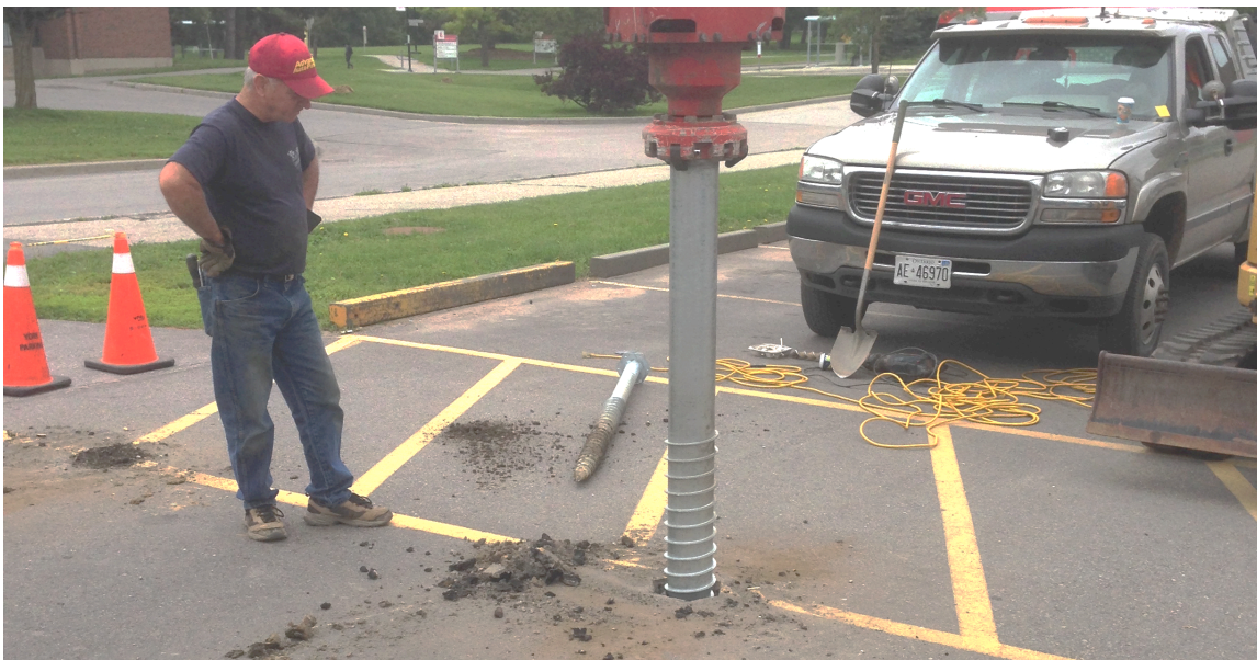
Figure 8: Drilling of the first ground screw. Photo Source: Mustafa Nazari
