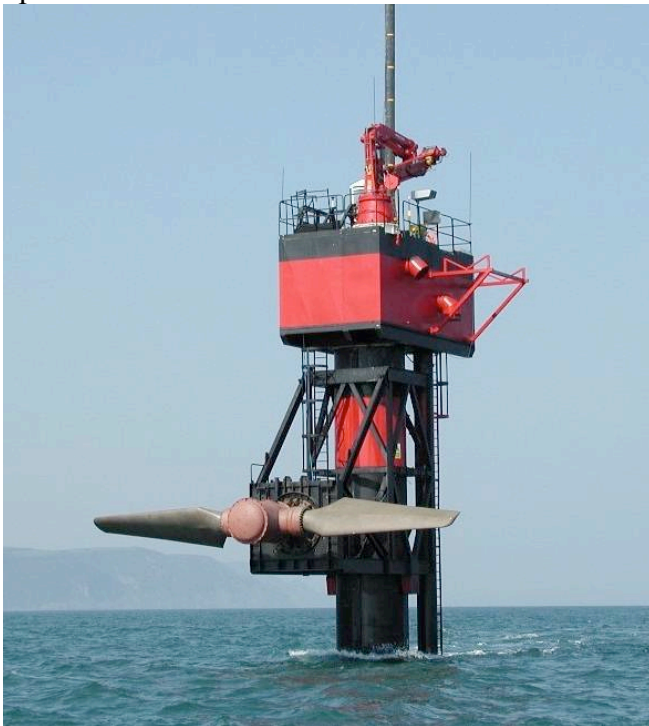
Figure 3: The SeaFlow tidal stream generator prototype with rotor raised" by Fundy/CC BY-SA 3.0
