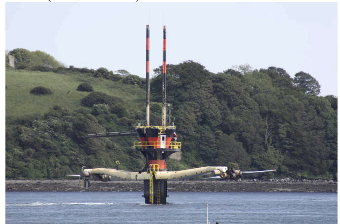
Figure 7: SeaGen tidal power plant, Strangford, County Down, Northern Ireland, 2011 (blades raised for maintenance)" by Ardfern/ CC BY-SA 3.0
