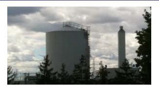
During the combined summers of 2010 and 2011, the tank stored 3,600 MWHRS(th) of heat recovery from CHP operations; which was then discharged to the community heat load at night.
