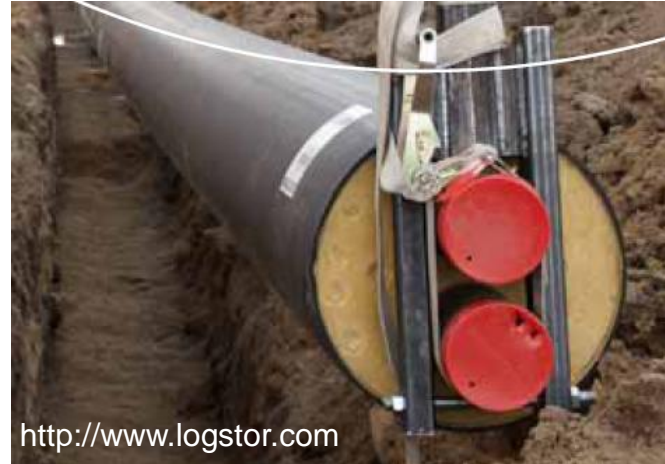
Innovative : Twin-pipe network
